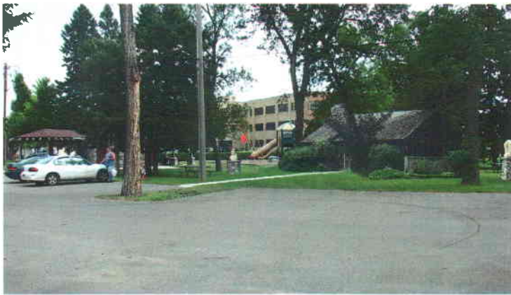
Cabin Facing North - Viewed from the Northwest
